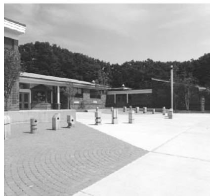
View of the brick pavers laid in a circular pattern with the decorative precast concrete bollards.
