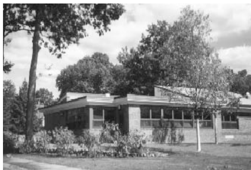
Under a phased construction schedule, work was completed while the building was occupied.
