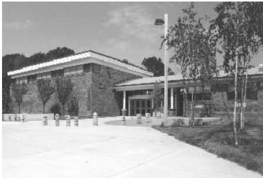
The Brown Elementary School was a composite project combining an addition to the school as well as major renovations.
